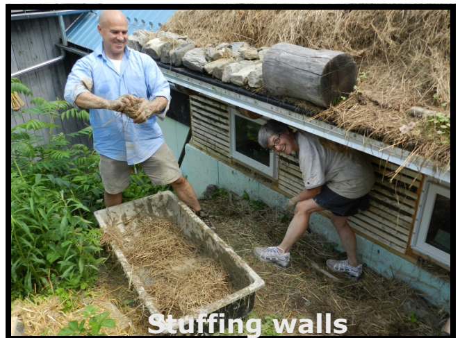
Mixing straw into clay slip
